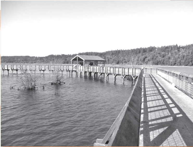
Above: A completed stretch of boardwalk over the restored estuary.
